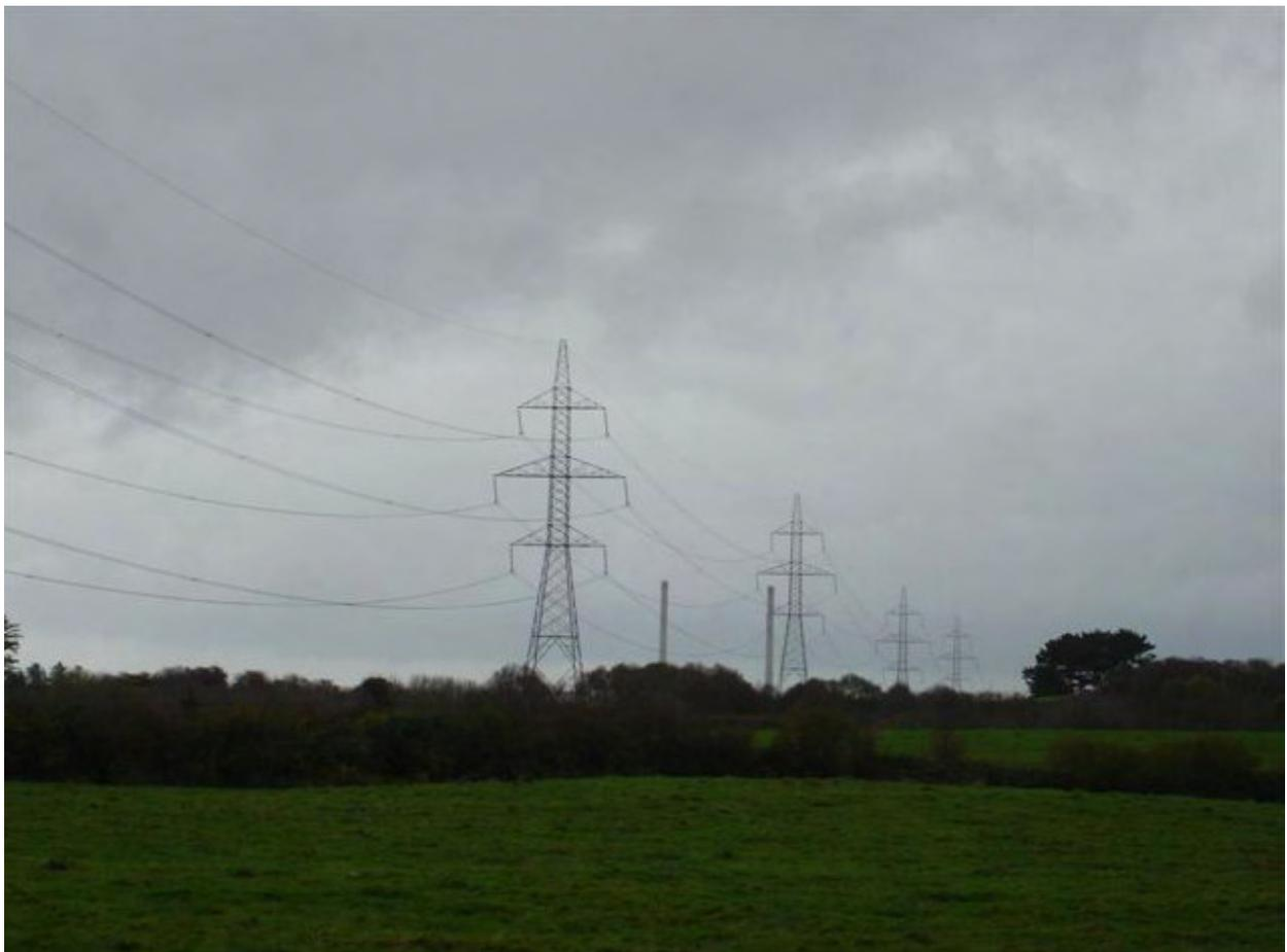
**Figure 2.20 400kV double circuit intermediate towers near Moneypoint generating station County Clare**
