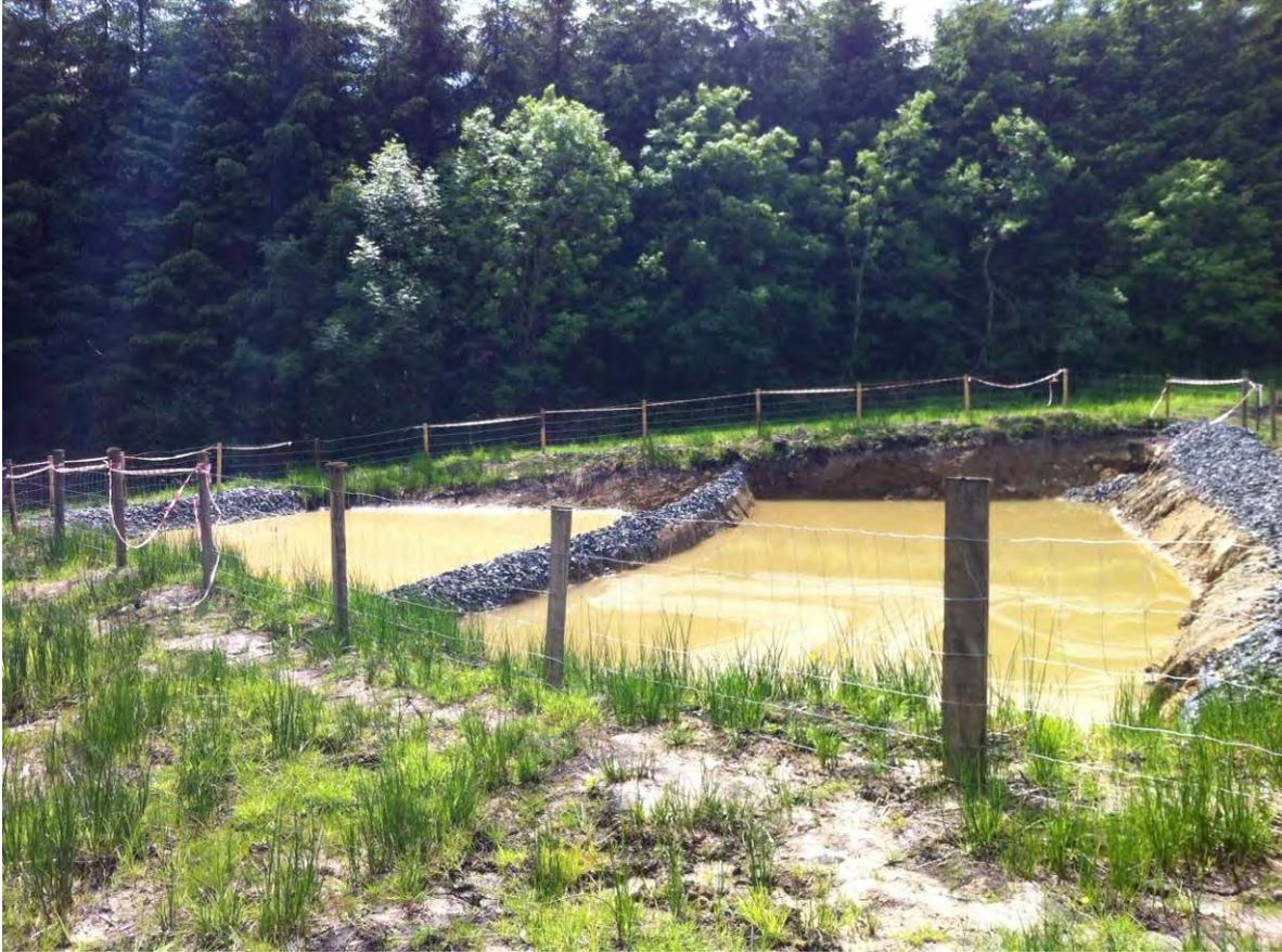
**Figure 2.12 Typical settlement/attenuation pond**
