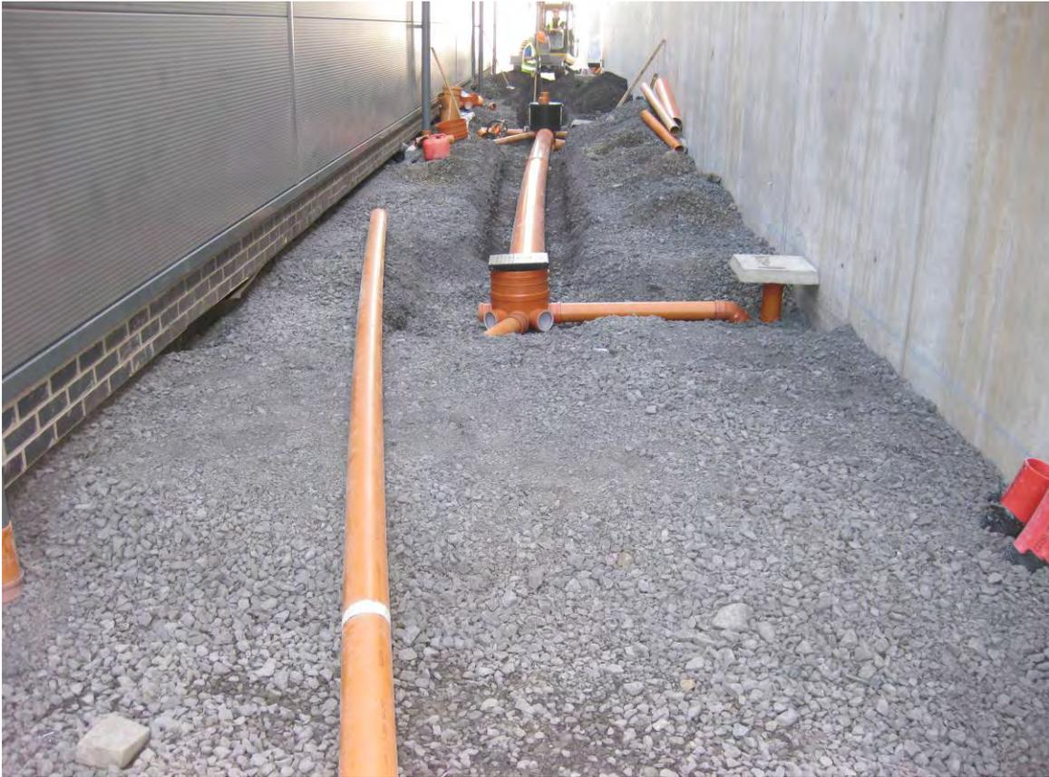
**Figure 2.19 Typical installation of drainage**
