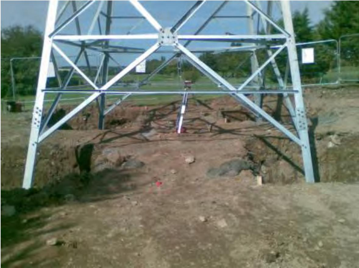
**Figure 2.28 Photograph of steel tower base in open excavations**
