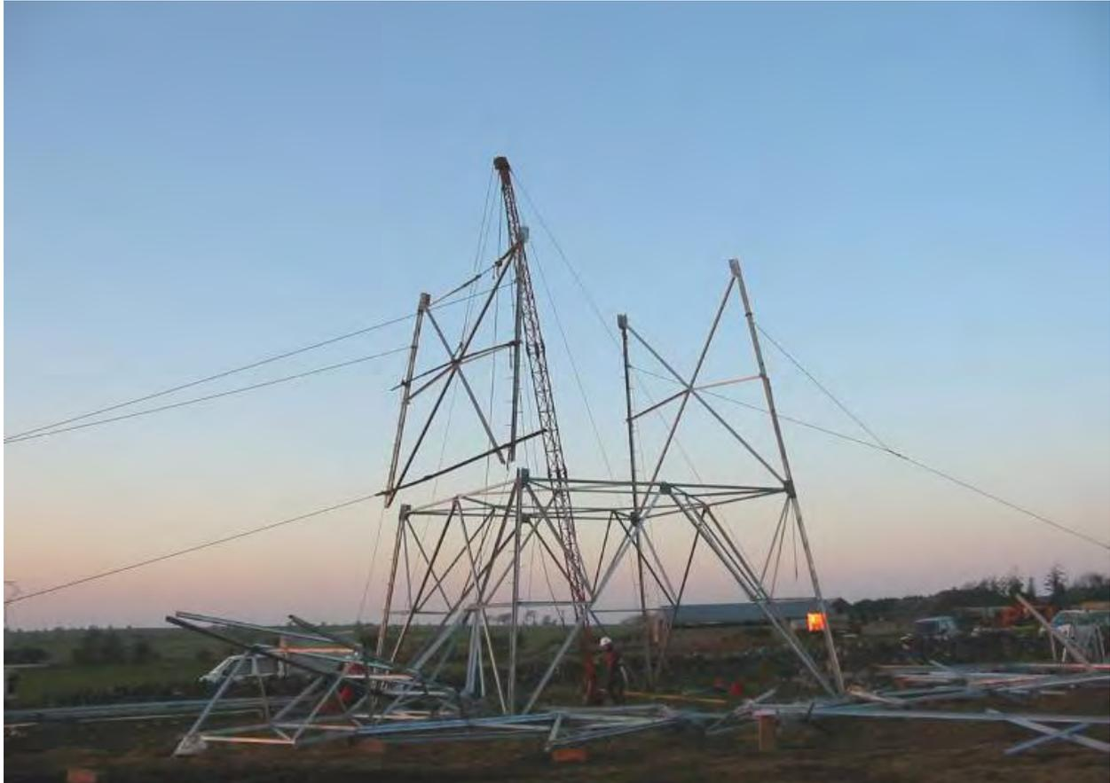
**Figure 2.23 Derrick pole at tower base**
