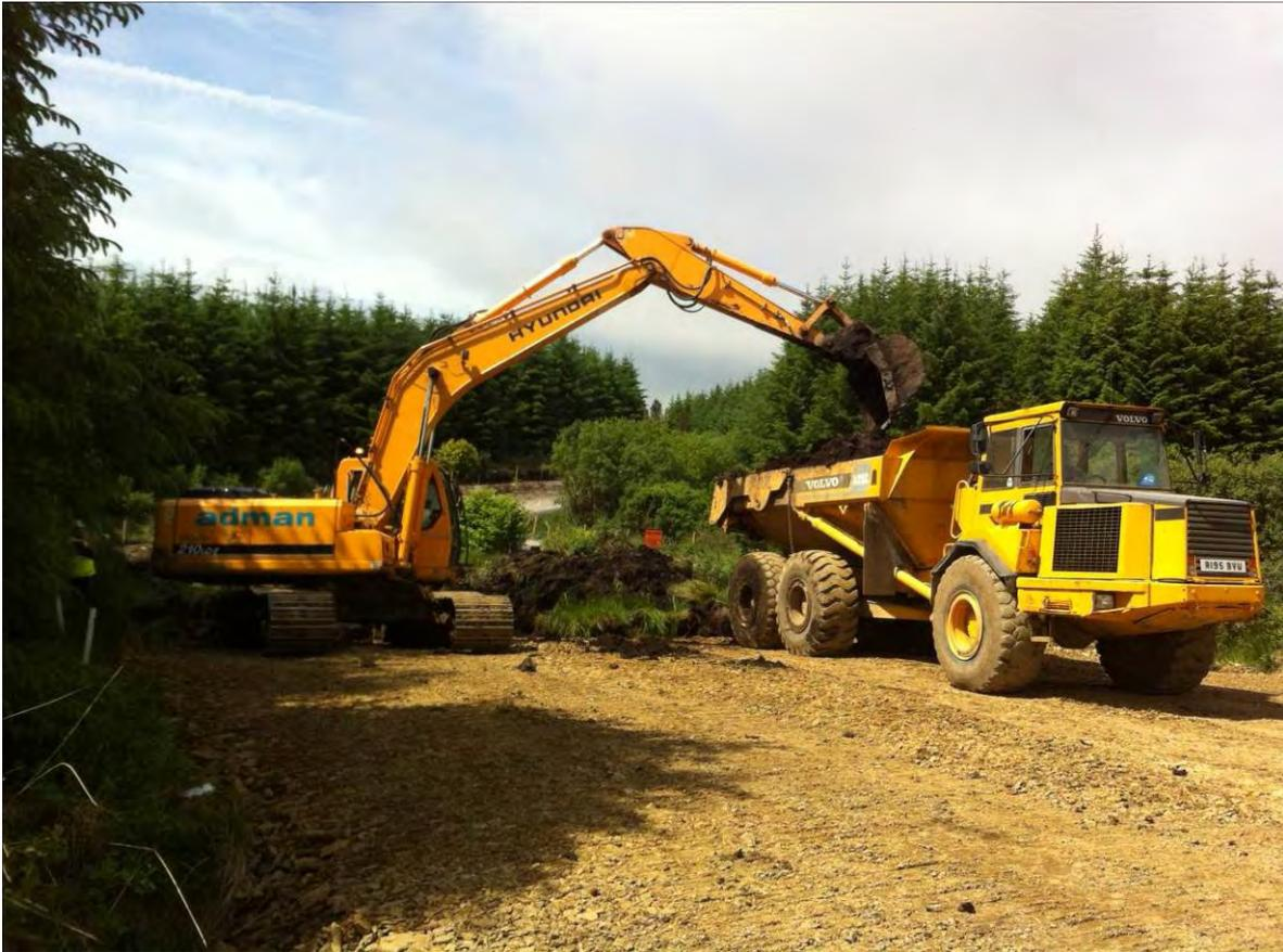
**Figure 2.13 Typical plant employed in the site clearance and earthworks phase of the project**
