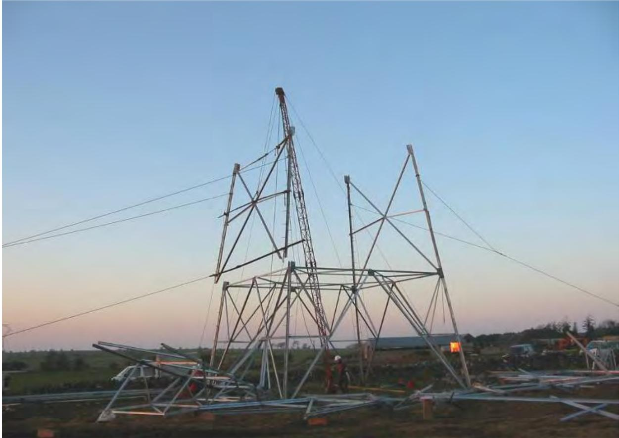
**Figure 2.23 Derrick pole at tower base**
