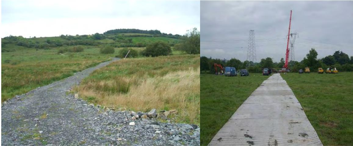
**Figure 2.35 Temporary Stone and Aluminium Panel tracks**
