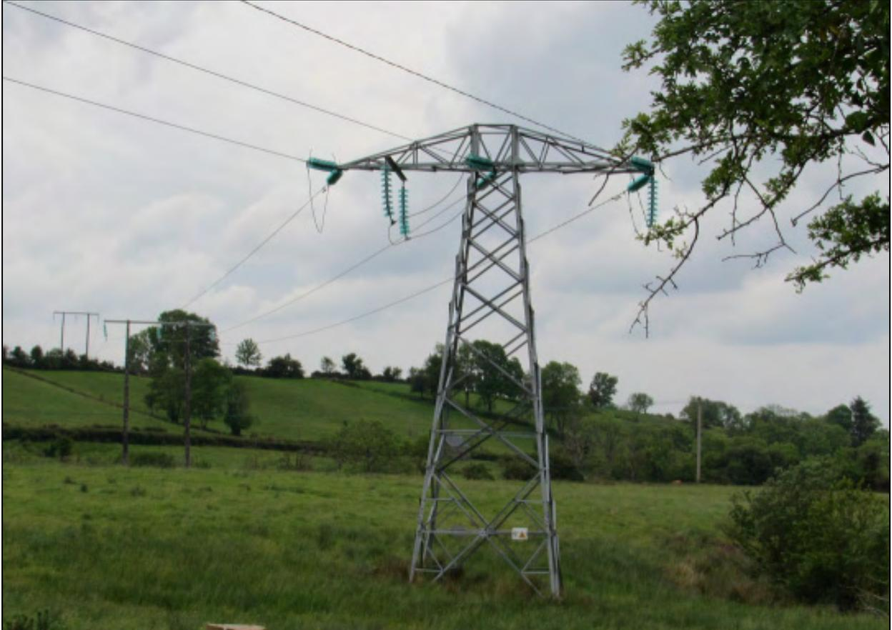
**Figure 2.9 Photograph of a 110 kV Non-Earthwire Angle Mast**
