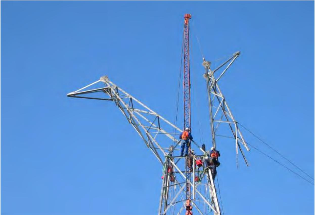
**Figure 2.24 Lower part of the tower head being dropped into position**
