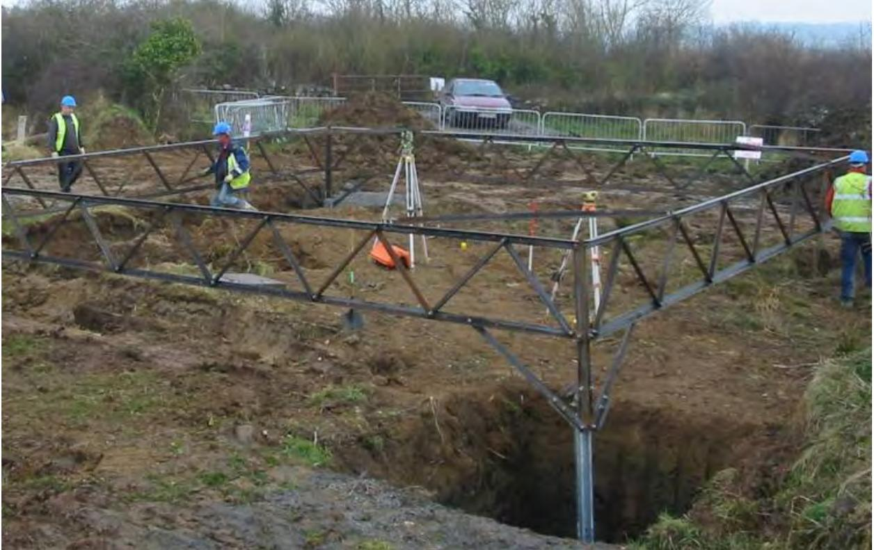
**Figure 2.22 Photograph of setting template being prepared for final concreting**
