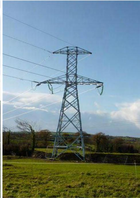
**Figure 2.27 Typical steel angle structure**
