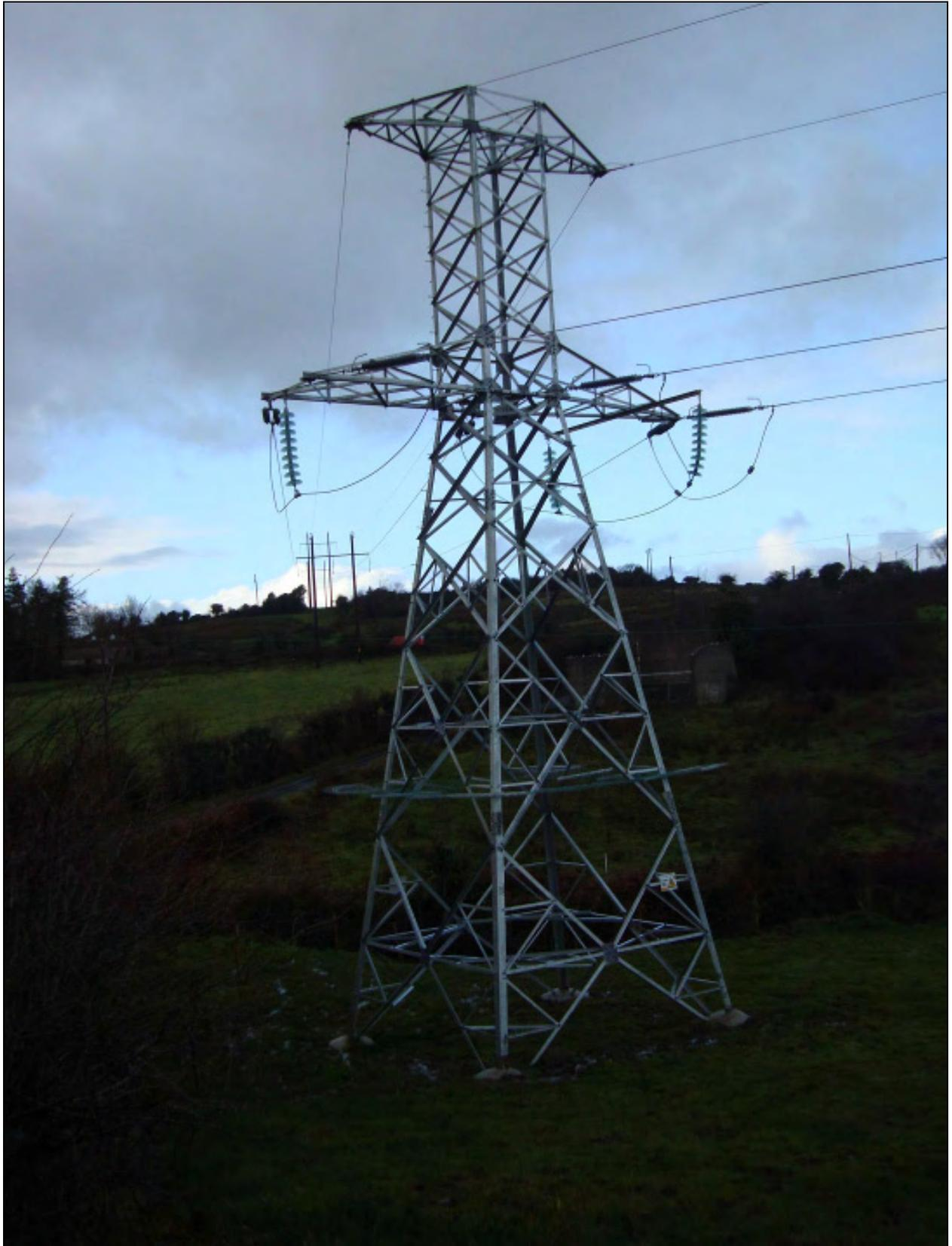
**Figure 2.7 Photograph of a 110 kV Earthwire Angle Mast**
