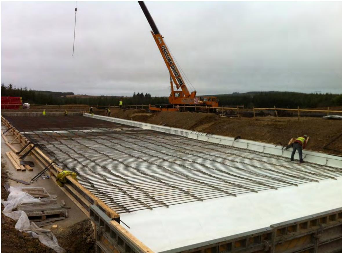
**Figure 2.14 Steel reinforcement fixing to foundations/ floor slab**
