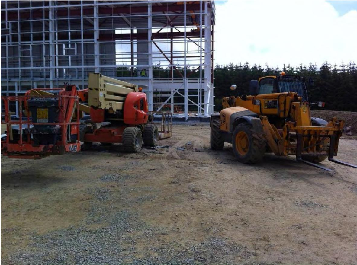
**Figure 2.17 Typical plant employed during building construction**
