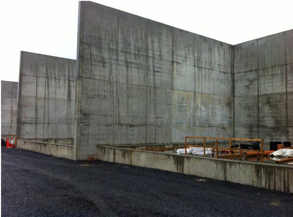
**Figure 2.18 Typical walled enclosures for transformers and shunt reactors**
