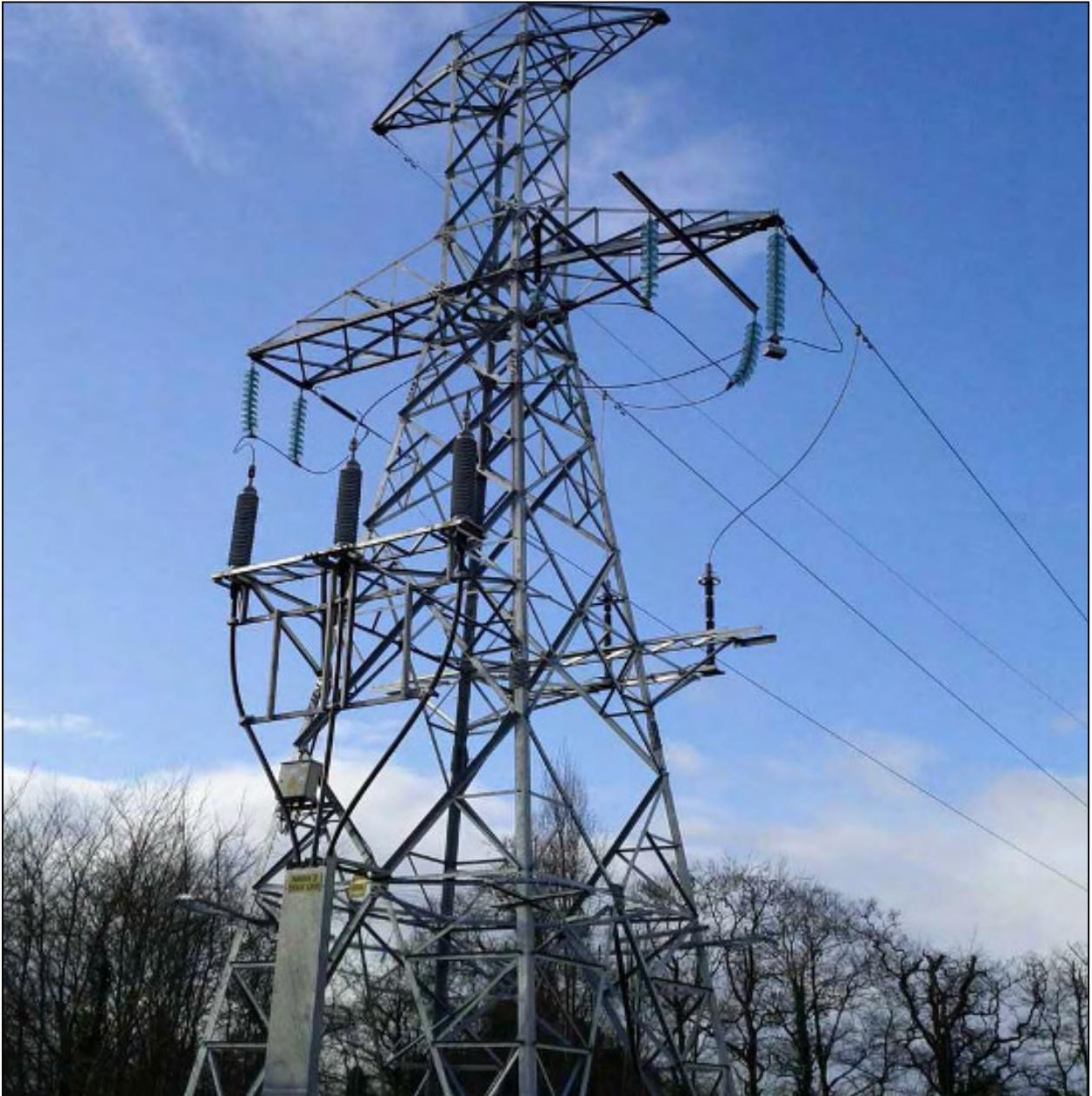
**Figure 2.4 Photograph of a 110 kV Earthwire Line/Cable Interface Mast**
