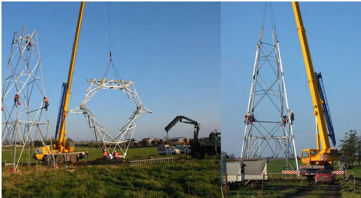
**Figure 2.25 Tower erection by mobile crane**
