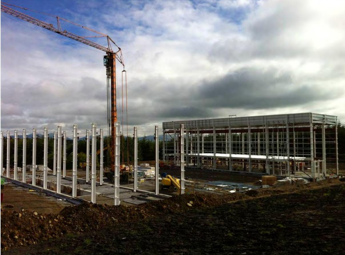
**Figure 2.15 Structural steel erection including bracing and gantry crane rail**
